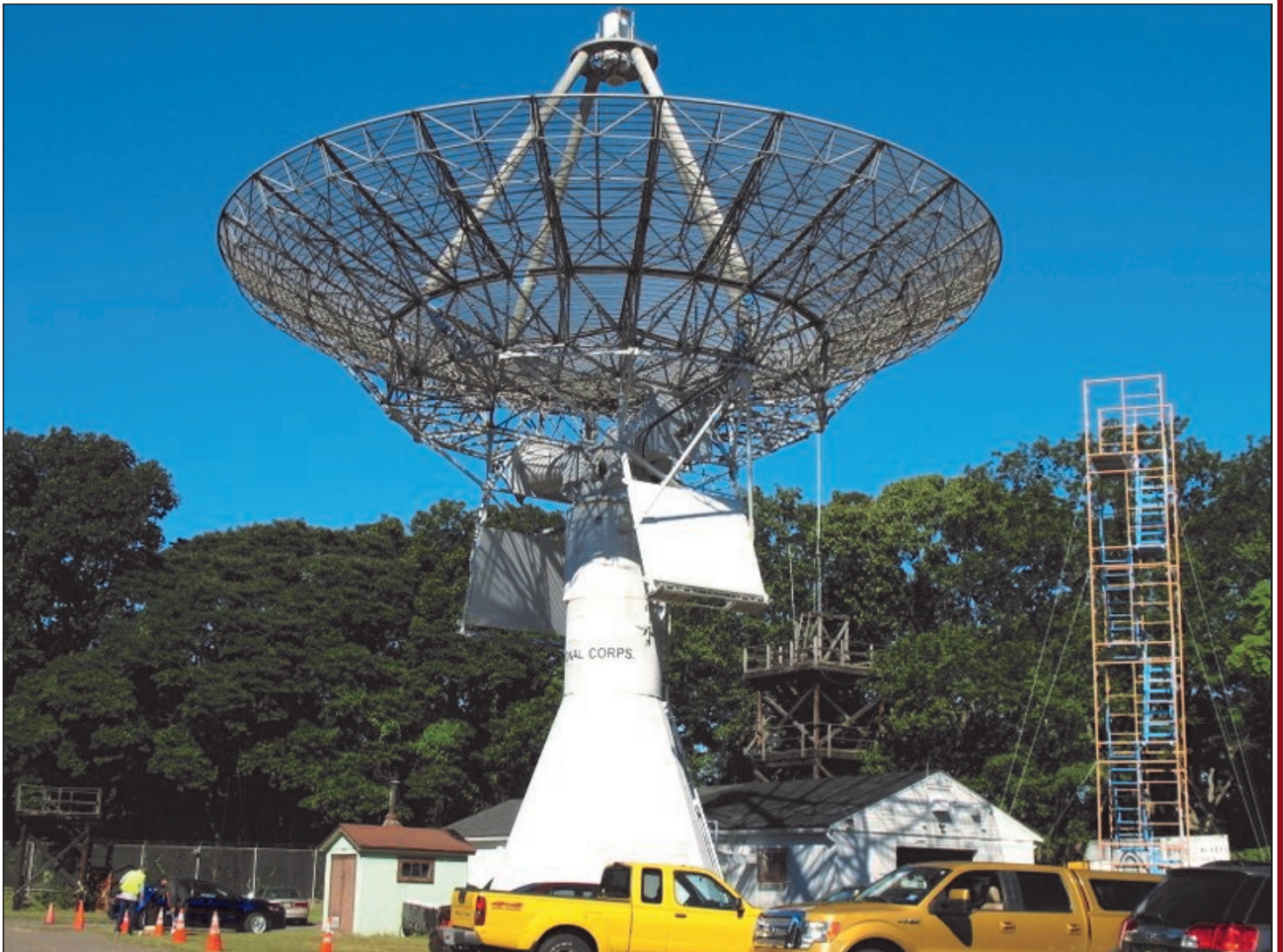
Note the tower to the right of the antenna, used for feed installation and maintenance
